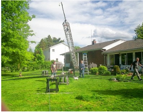
Beam resting on saw horses prior to lifting into position.
