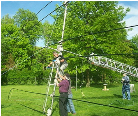
Attaching antenna to mast.
