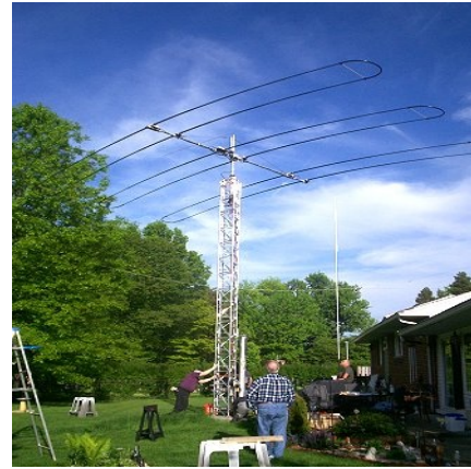
Success! Antenna & tower raised into position.
