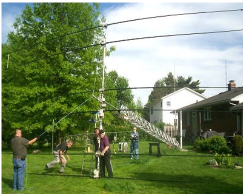
Antenna mounted on mast. Ready to raise into position.
